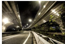
ROADS AND INFRASTRUCTURES
